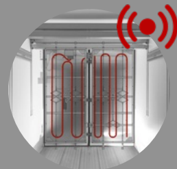
Loop cable inside the frame
